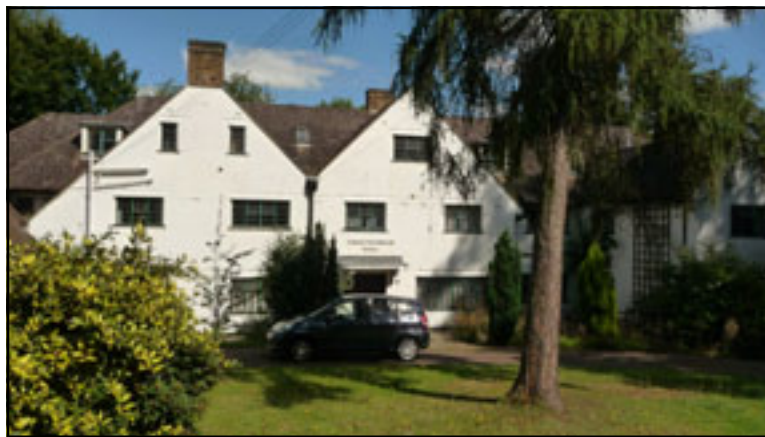
South west elevation of Troutstream Hall
