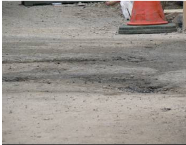
Examples of deterioration and patching to footways
