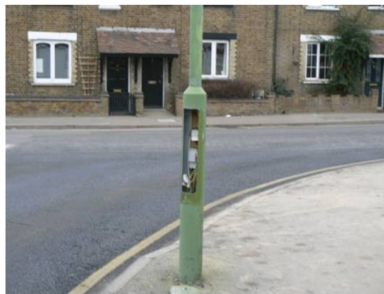
Example of deterioration to street lighting
