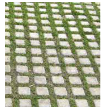
Figure 91: Permeable concrete paving.
