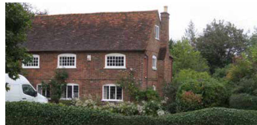
Green End Farmhouse - red brick façade with upper floor horizontal sliding sash windows and ground floor multi-paned casement windows with cambered heads.
