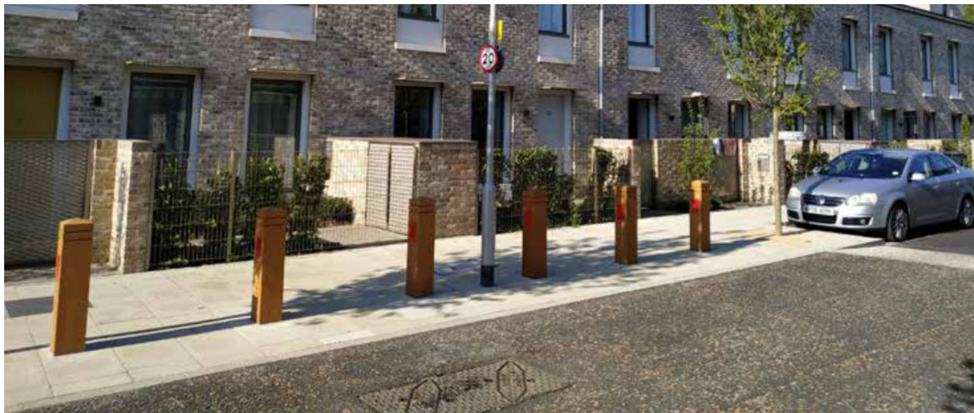
Figure 44: Example of a raised mid-block pedestrian crossing on a 20 mph street on Goldsmith Street, Norwich (note: many councils require blister tactile pavers at crossings to guide visually disabled pedestrians).
