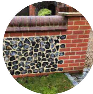
Knapped flint and red brick boundary wall
