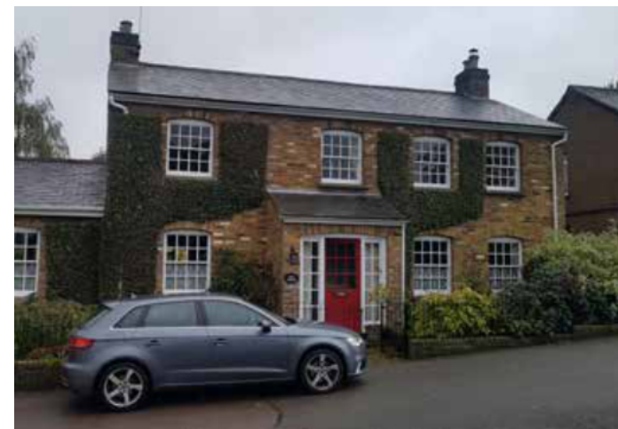
Figure 7: Yellow stock brick and slate roof building with recent porch addition.
