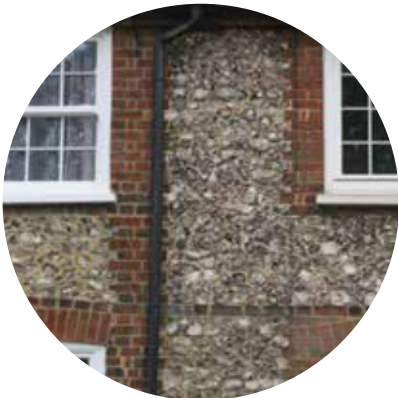
Red brick trim and knapped flint infilling
