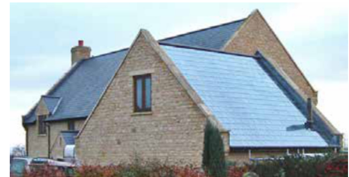
Figure 84: Integrated design for solar panels.
