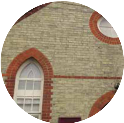
Red brick trim and yellow brick infilling
