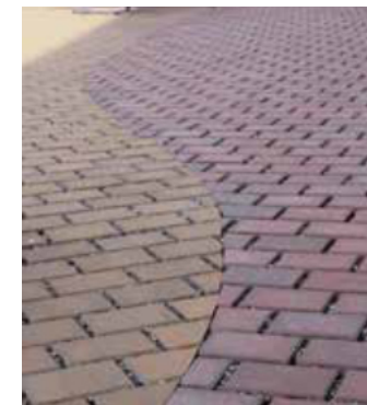
Figure 90: Permeable brick paving.
