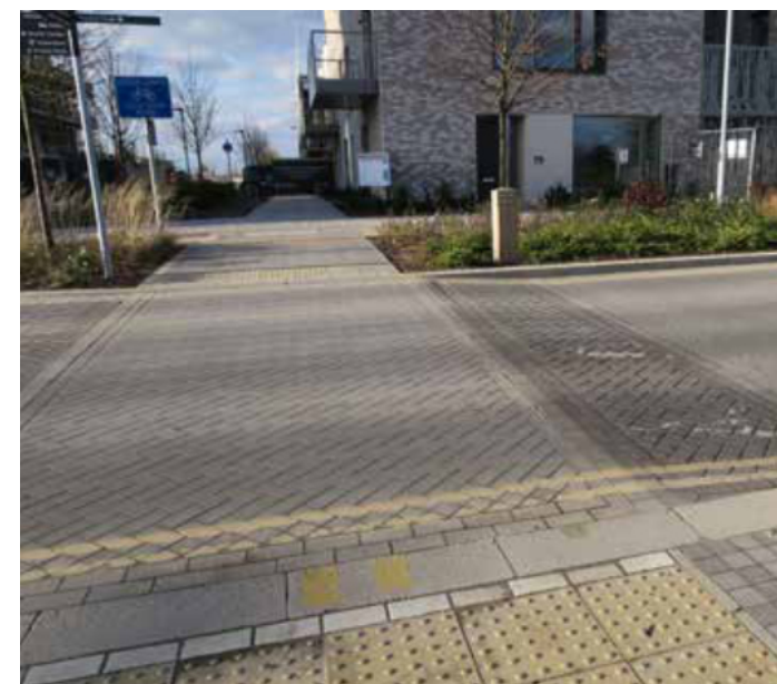
Figure 45: Example of a raised crossing across a main road in Cambridge, with contrasting paving materials and space for low-level planting and street furniture (note: traditional paving materials and muted colours are often preferred in conservation areas).
