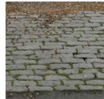
Granite block vehicle crossover
