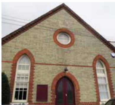
Former Providence Mission Hall with bicolour brickwork around openings.
