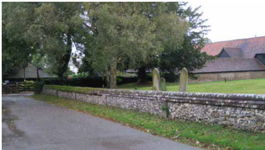
Figure 72: Church yard wall built with local flint.
