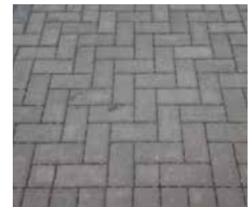
Dark grey concrete block paving
