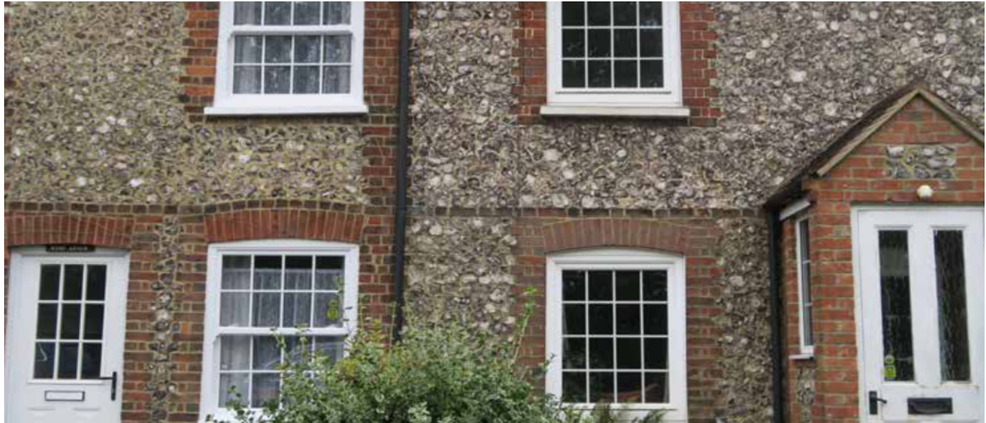
Figure 69: Façades with consistent arrangement of multi-pane windows with attractive brick ornamentation and articulations.
