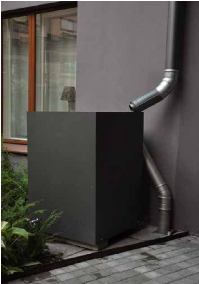
Figure 87: Examples of tanks used for rainwater harvesting.
