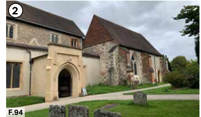
Figure 94: St Lawrence Church, an Anglican church on the High Street
