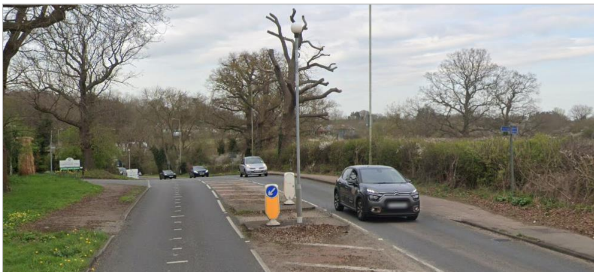
Image 2.14: Uncontrolled pedestrian crossing on Oxhey Lane
