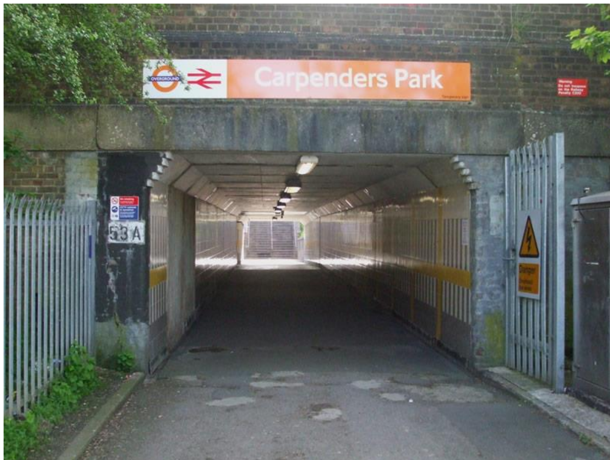
Image 2.29: Station Entrance and Underpass
