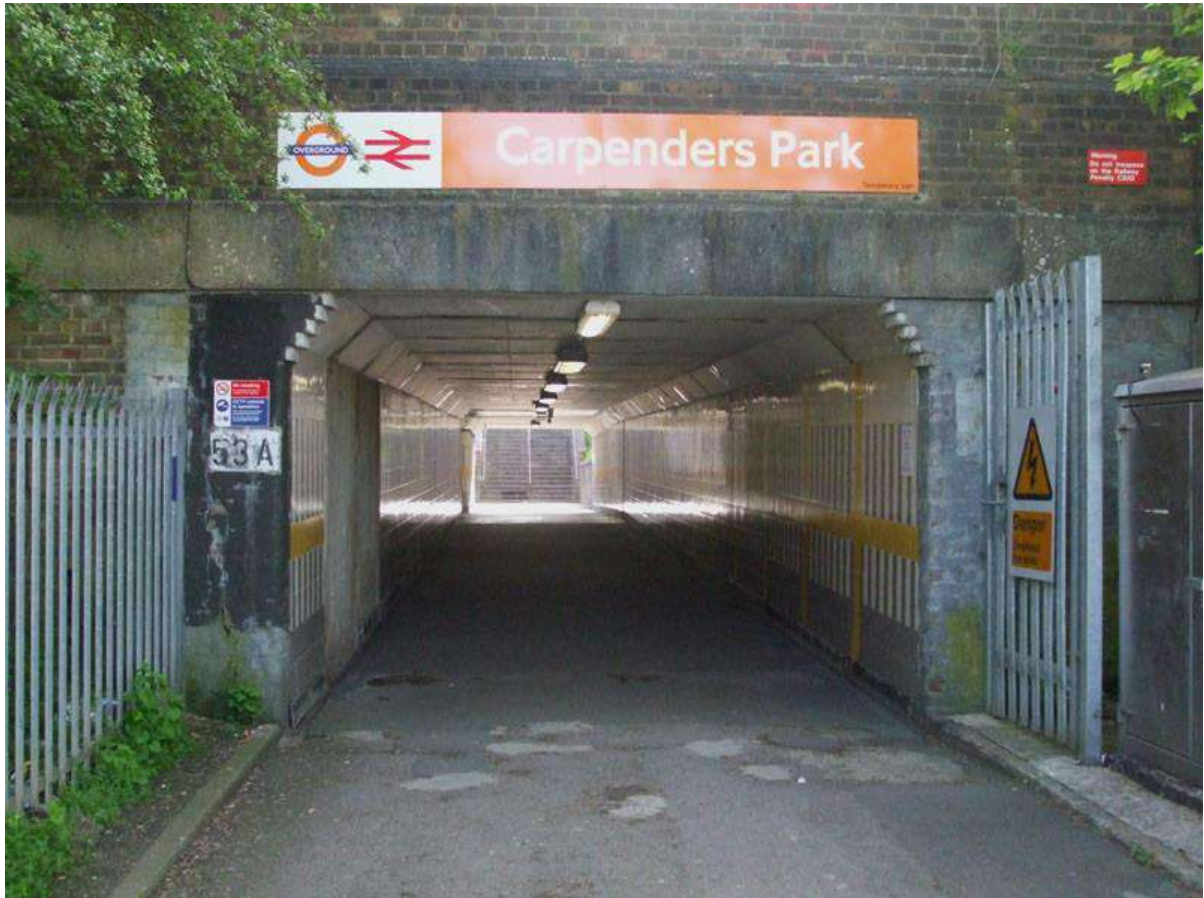
Image 2.29: Station Entrance and Underpass
