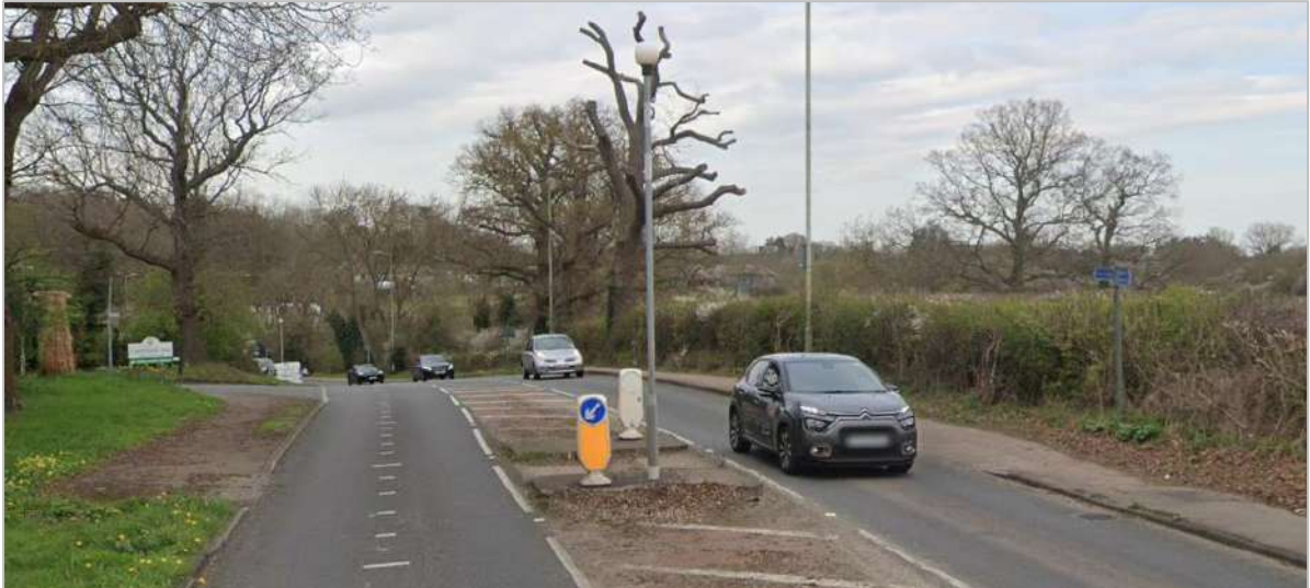
Image 2.14: Uncontrolled pedestrian crossing on Oxhey Lane
