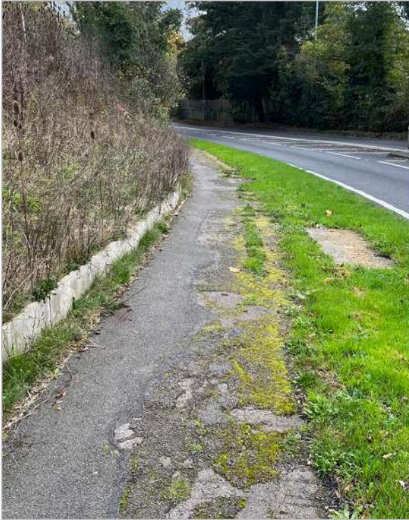
Images 2.3 and 2.4: Footway on Oxhey Lane (looking south)
