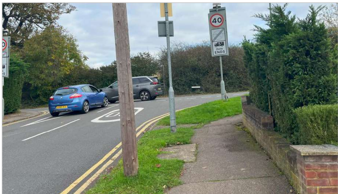
Image 2.8: Footway at junction (looking east)
