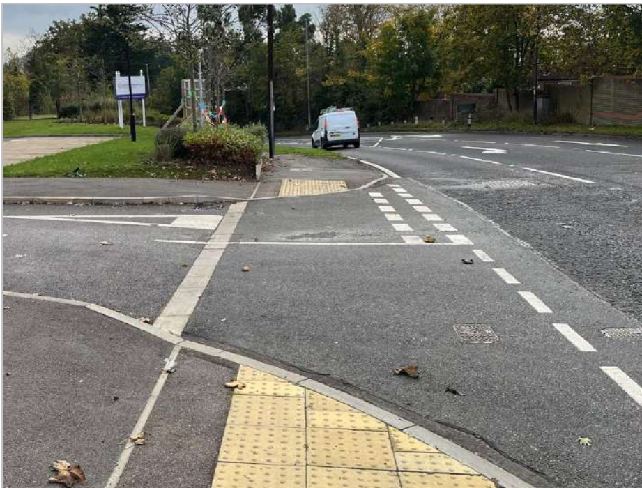
Images 2.4: Crossing at Carpenders Park care home access
