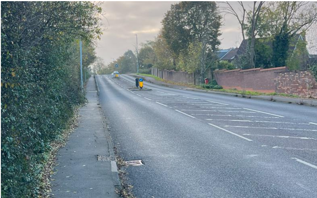
Image 2.1: A4008 Oxhey Lane (looking south) along site frontage
