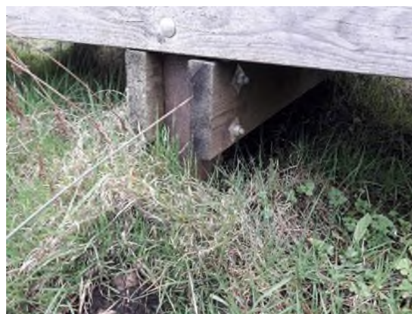
Existing boardwalk construction detail
