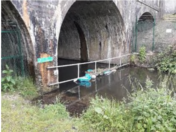
Barrier at western end of site
