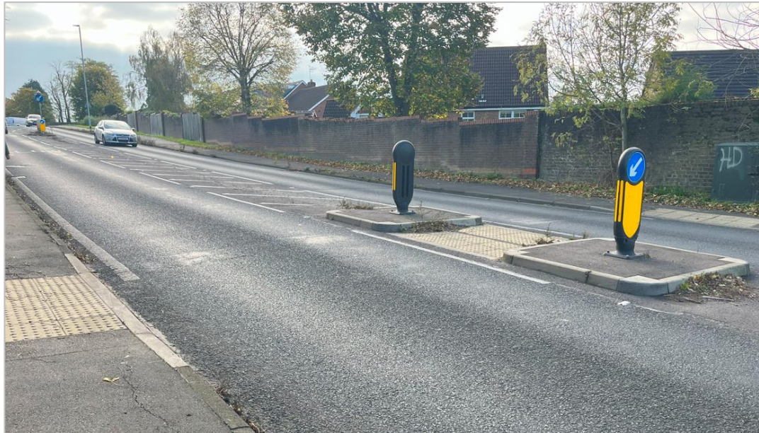
Image 4.1: Pedestrian Crossing Oxhey Lane
