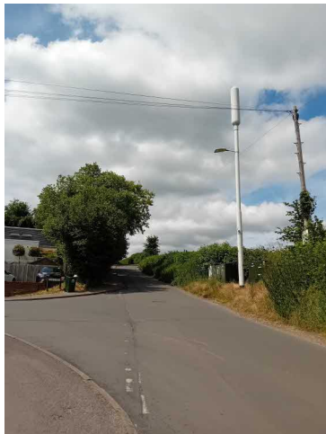
Photo 4— Overhead services and cabinets on Little Green Lane
