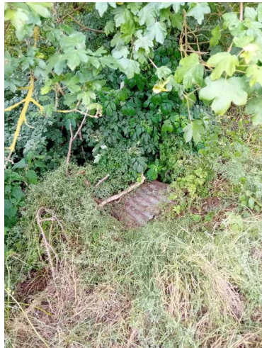
Photo 16— Evidence of waste materials in the pit
