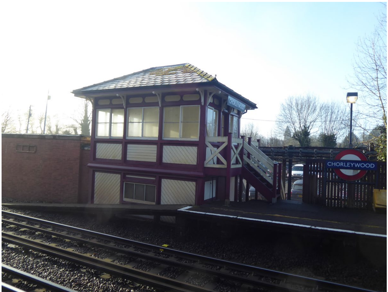
Figure 17 View of signal box from north platform
