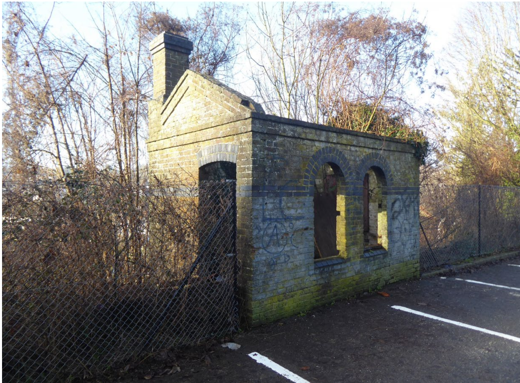
Figure 10 View of nineteenth century former railway building in car park
