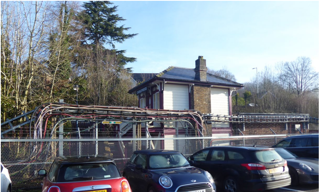
Figure 18 View of signal box from car park
