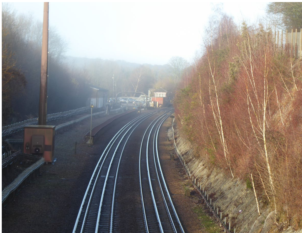
Figure 19 View of signal box from Chorleywood Bottom Bridge
