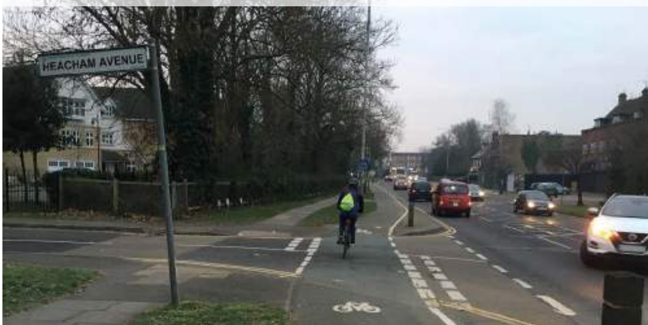
Figure 10.16: Partial set back, marked priority crossing, Hillingdon
