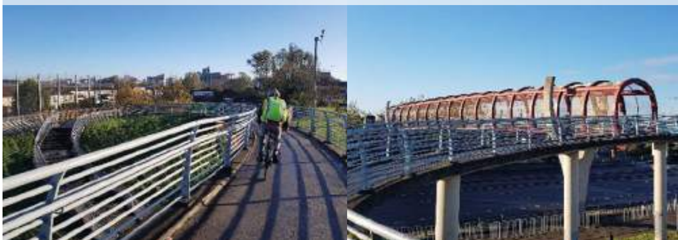
Figure: 10.53: Overbridge with curved ramp approach, Belfast
