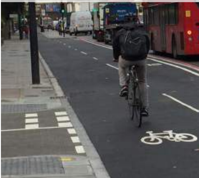
Figure 7.10: Tight kerb radii at residential side street
