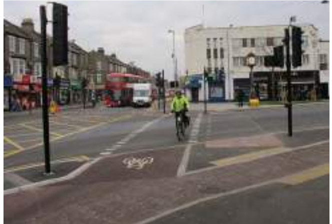
Figure 10.26: Circulating Cycle Stage Junction, Waltham Forest
