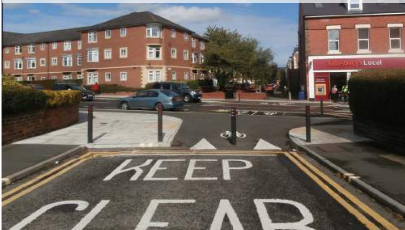
Figure 8.5: Cycle route crossing a footway, Newcastle
