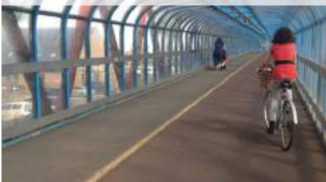
Figure 10.50: Covered pedestrian/cycle bridge across railway tracks, Cambridge
