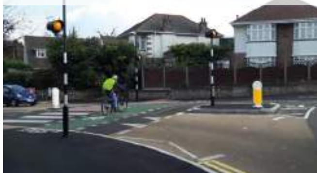
Figure 10.38: Roundabout with parallel crossings and shared use paths, Bournemouth
