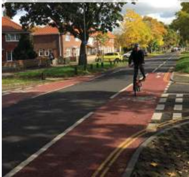
Figure 6.21: Centre line removal, Norwich
