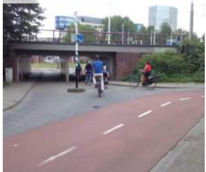
Figure 10.48: Cycle and pedestrian route grade separated from carriageway, Arnhem, Netherlands
