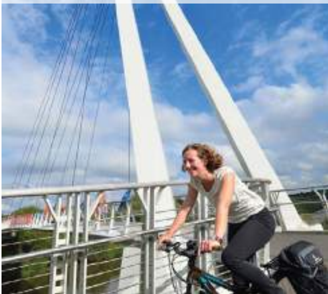
Figure 10.49: Diglis Bridge, Worcester
