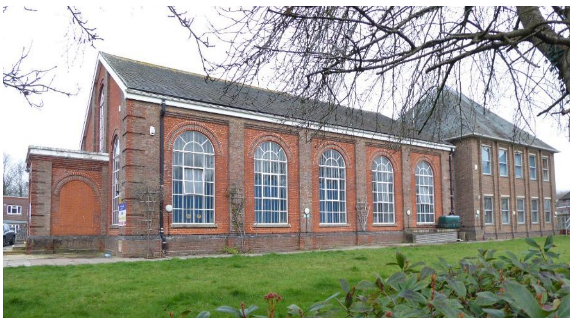
Figure 22 South elevation of 1930s pump house building and later addition.
