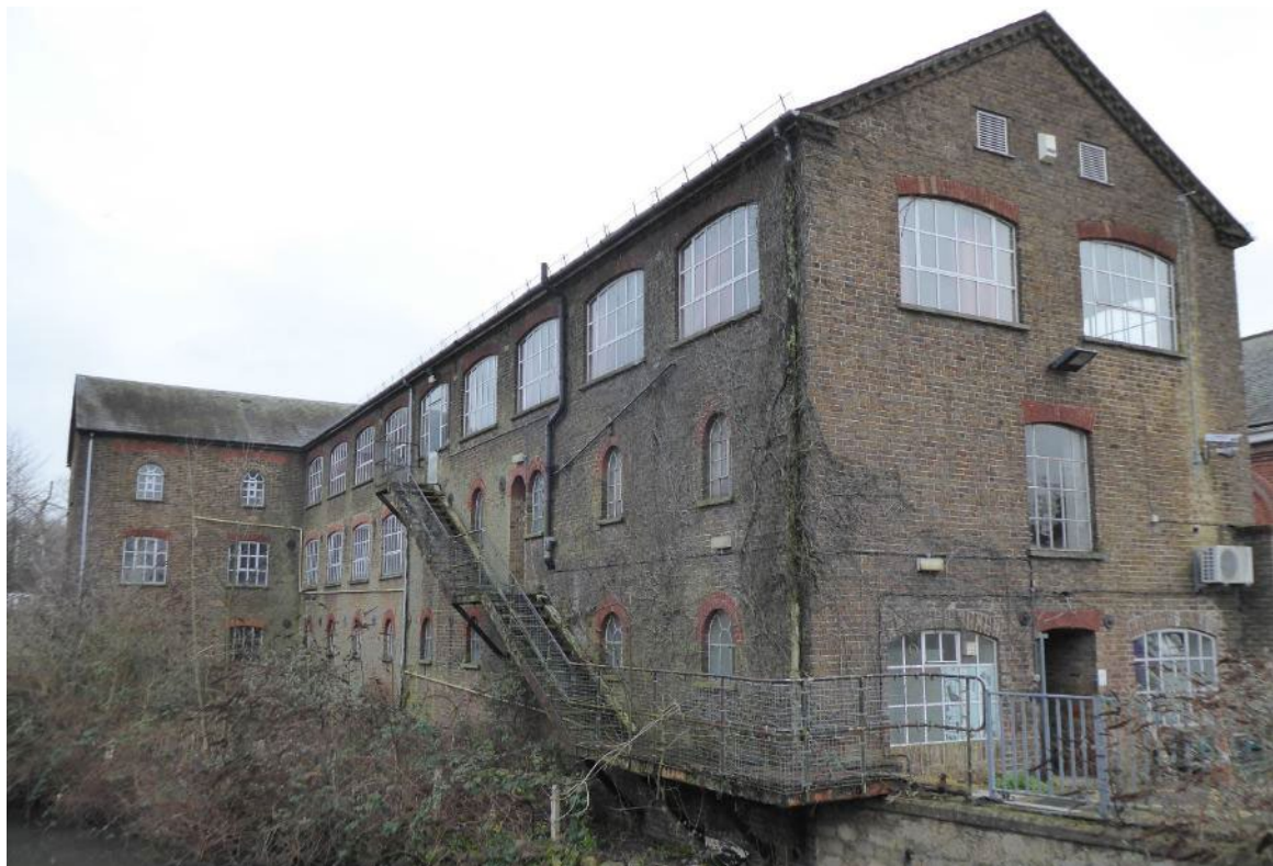
Figure 20 North and east elevations of the nineteenth century former mill building, later repurposed as a pump house.
