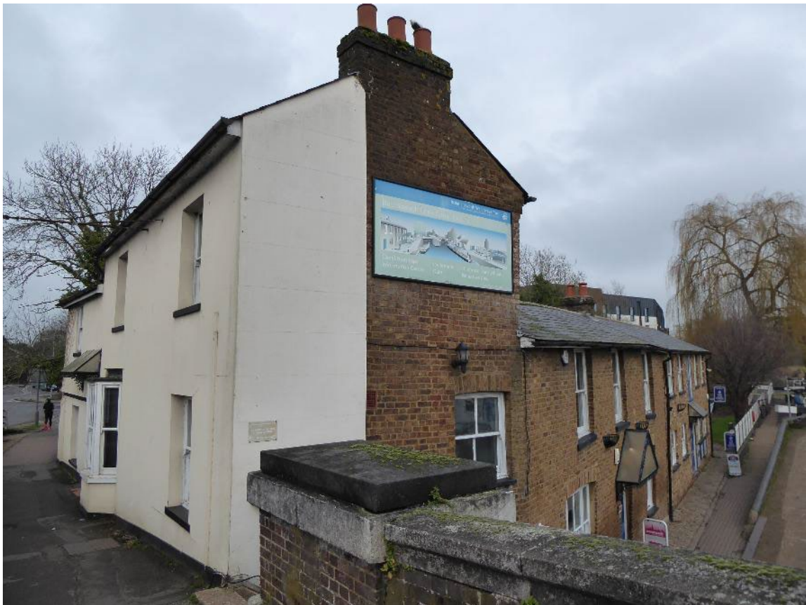
Figure 26 South elevation of 99 Church Street.
