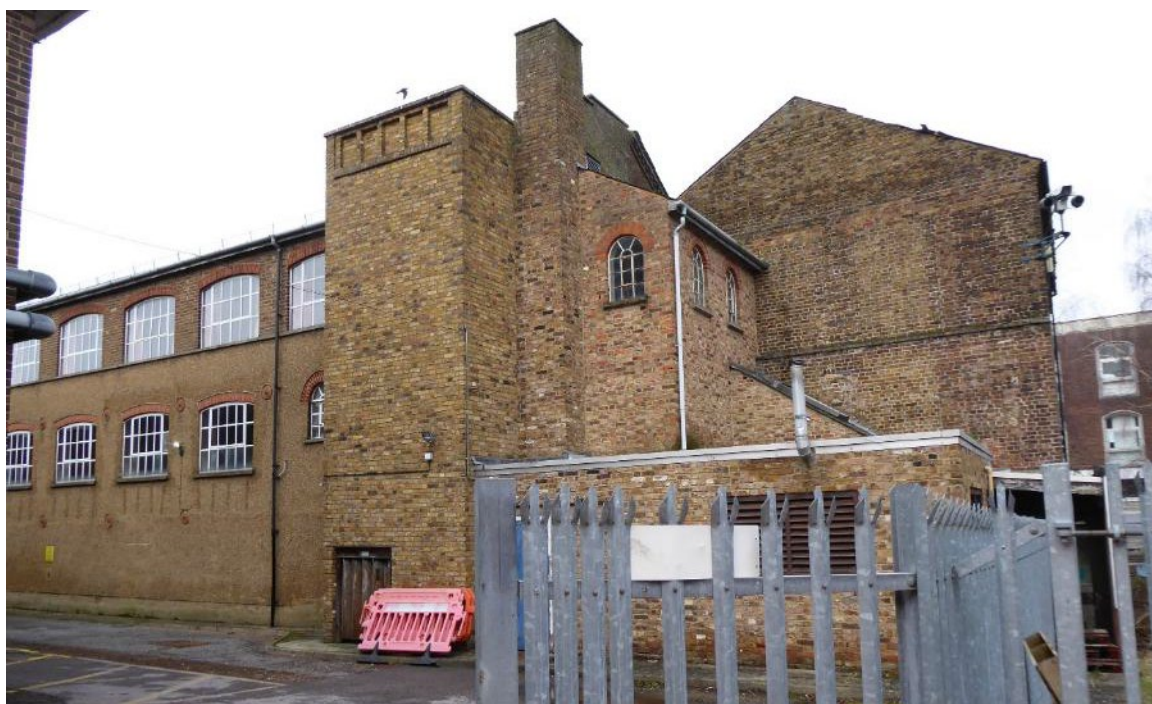
Figure 21 South elevation of the former mill building.
