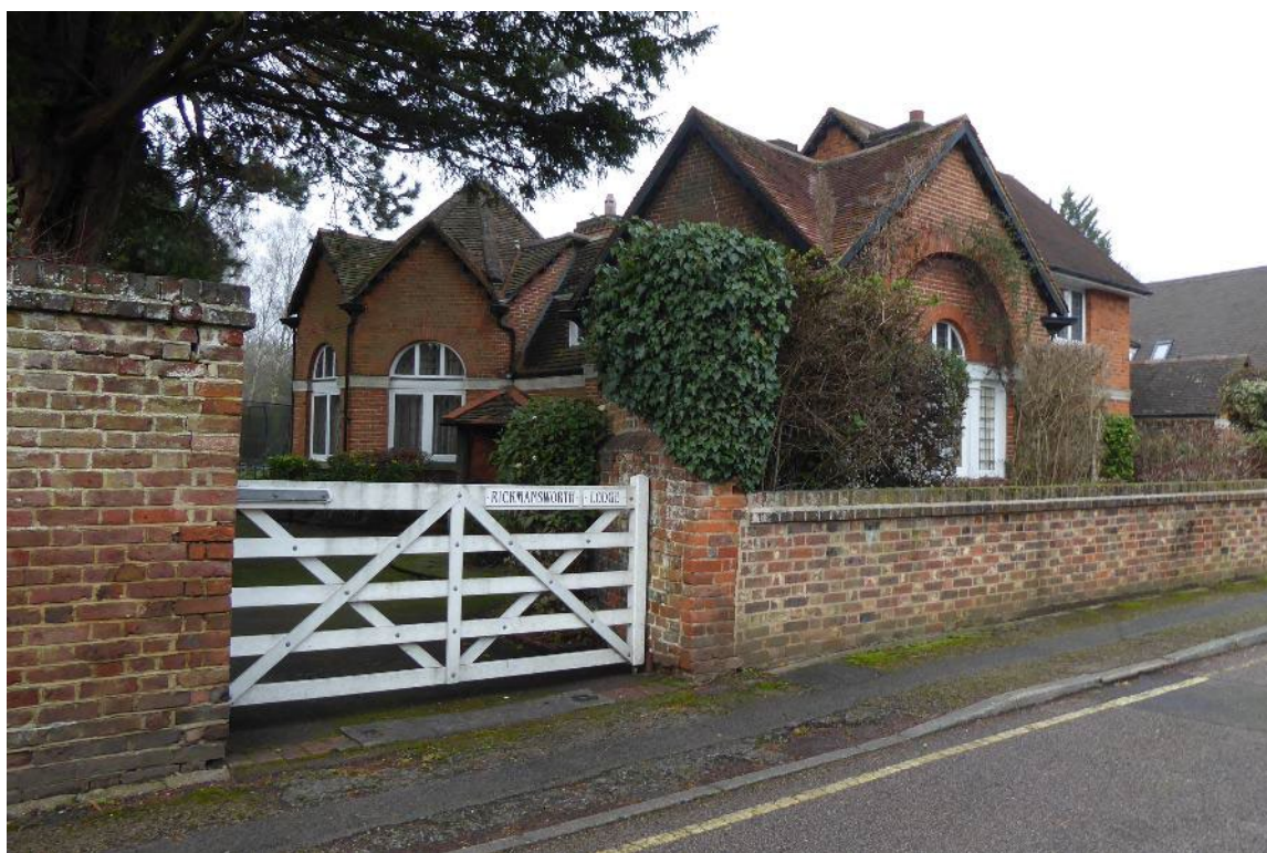
Figure 31 West and south elevations of 17 Moor Lane.
