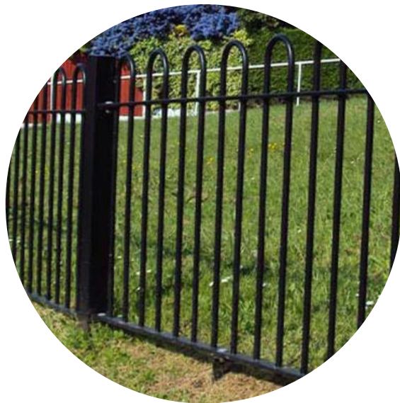
Example of bow top fencing to be used in the medium risk area
